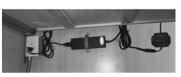
the cupboard. Often, there is an excess supply of wire provided so keeping the wires out of the way of normal activity is suggested. Peel the clear release liner off one half of the velcro patches and stick it onto the cabinet wall. Secure the wires using the mating velcro piece. If the velcro patches do not stick to your cabinet wall, use the strap included. Cut the strap to the desired length and drill the screws into the cabinet wall to secure your transformer and access cords.
