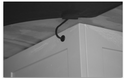
Cable hole after finishing plug is installed.
