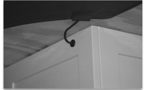
Cable hole after finishing plug is installed.
